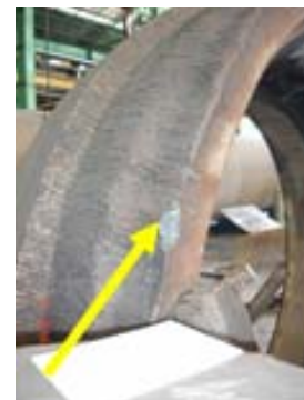
Gambar-1 Posisi pengambilan sampel Roller tyre Gagal (RTG)
