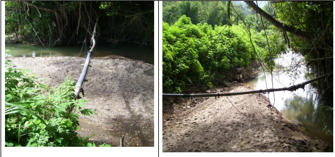
Picture 2: Piping irrigation water to the neighboring sub-village (Salo).
