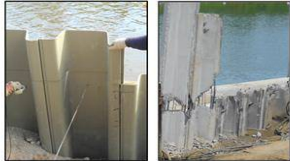
Figure 12 Cutting off vinyl and concrete sheet piles
