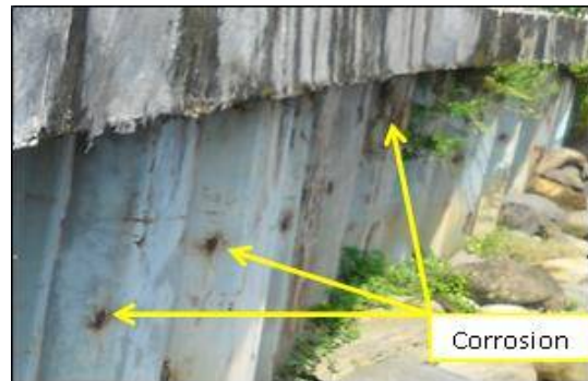
Figure 13 Corrosion on steel sheet piles
