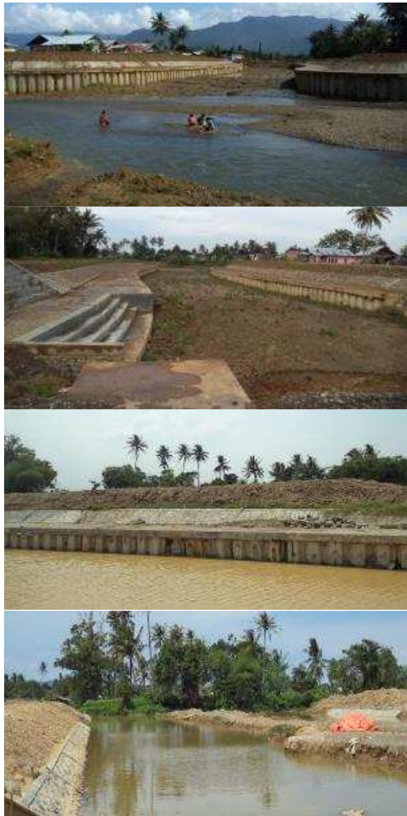
Figure 4. Luruih River normalisation project
