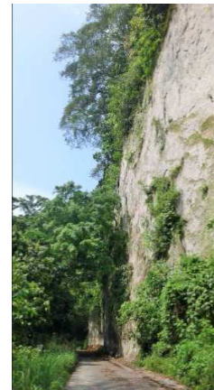
Figure 1. Sianok Canyon wall can stand up to 90° the township above the Sianok Canyon are now in a very dangerous situation where the distance between the building with the edge of top side of the Canyon wall just in a matter of less than 5 meters. The investigation on this area is needed to reduce the disaster risk as it has happen in the other place (Hakam et al, 2013).
