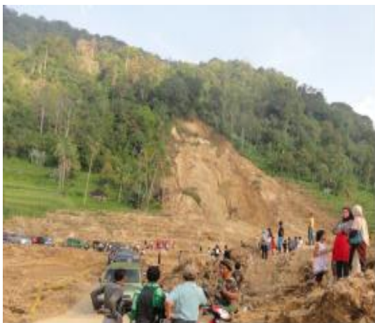
Figure 8 Maninjau – Agam Landslide in 2013 (Hakam et al, 2013)
