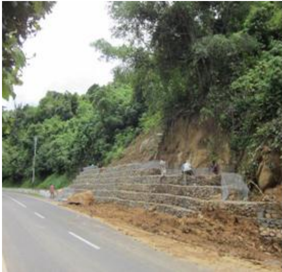
Figure 7 Remedial action using gabions
