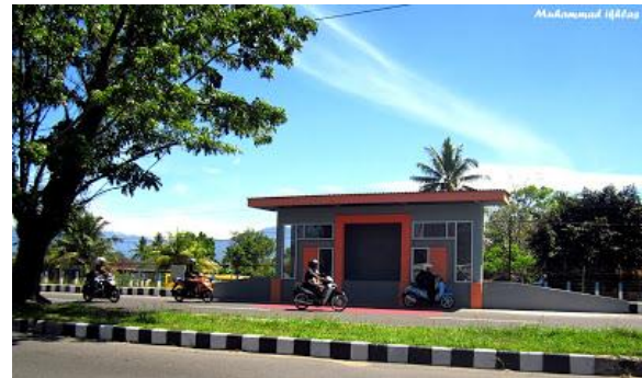
Figure 4 Trans Padang Metro Bus Stop facility
